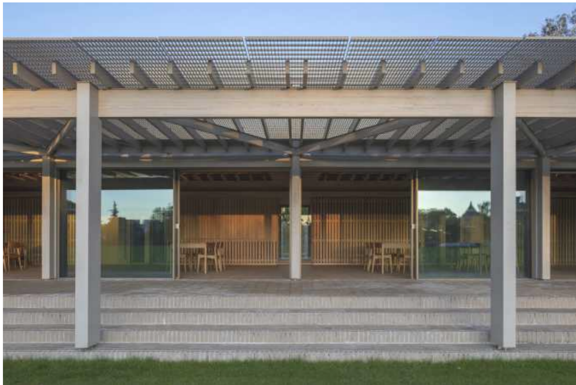
Sports Pavilion - Niall McLaughlin Architects
